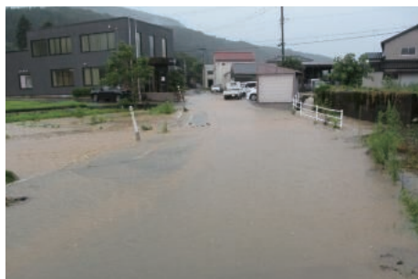
Kawachimachi Fukuoka Due to debris flow in the irrigation water, flooding occurred in fields and on roads.
